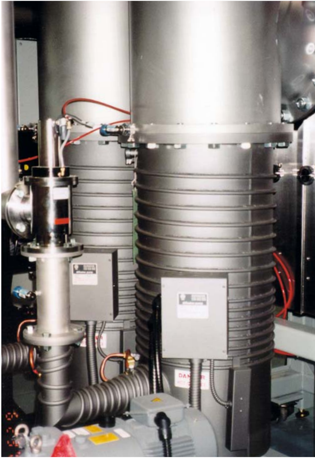
Courtesy of Mill Lane Engineering
